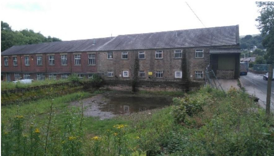
A 2016 view from the NE again shows the likely 1831 stonebuilt portion of the mill. Its windows abutted directly under the eaves/guttering in the fashion characteristic of that time. The slate roof at that date was possibly not the original.
