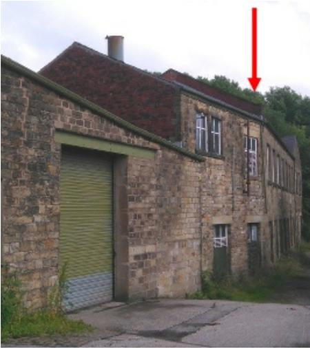
The west face of the mill had a very clear building break, (indicated by the arrow). The portion of the mill to the right of the break was built from a much better quality of stone, quite carefully dressed almost to ashlar standards, with good quality lintels and sills reflecting improvements in quarrying techniques achieved by the time that this section was erected. It probably postdated the 1847 Ordnance Survey map, perhaps comprising a later stage of development.
